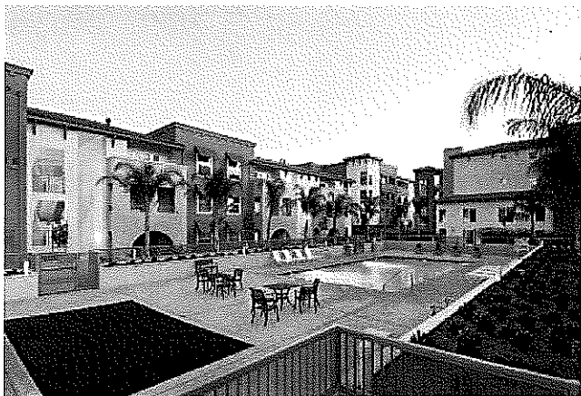
Corde Terra Village (Courtesy of ROEM Corp.)
